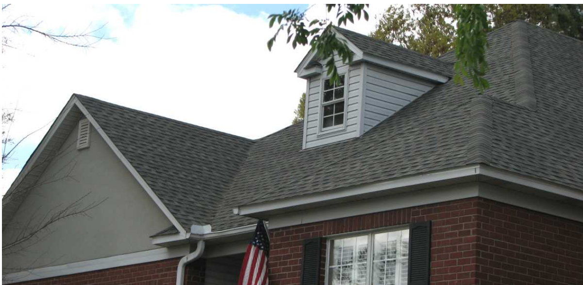
Nabors have a new roof
