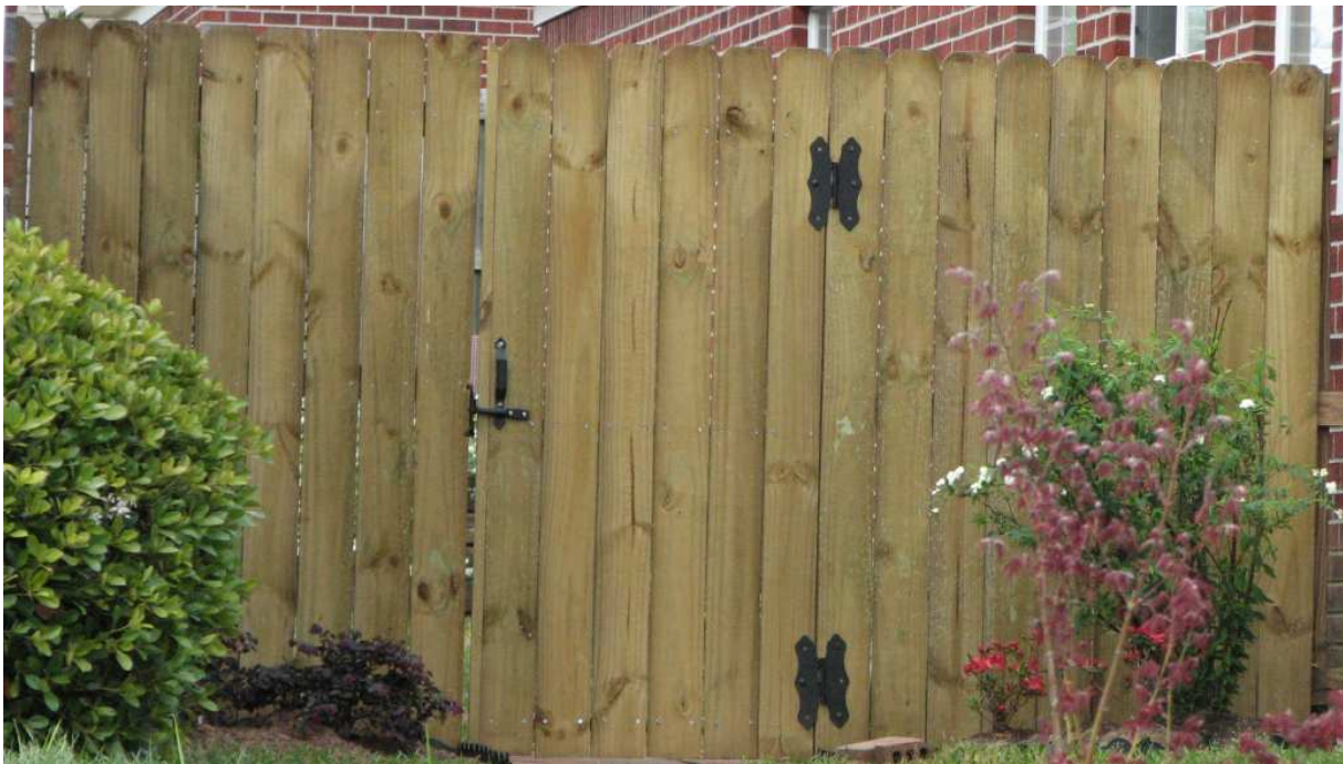
Front portion of fence built by Charles Snyder between the Snyder and Shumacher homes
