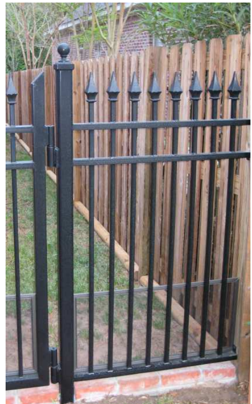
RIGHT: New paint for the Spence and Drury ironwork fence
